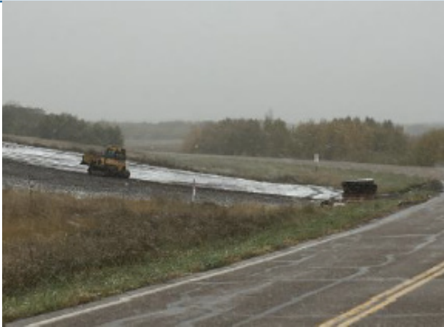
Dozer packing subsoil – SF 32 – Sept 21, 2018
