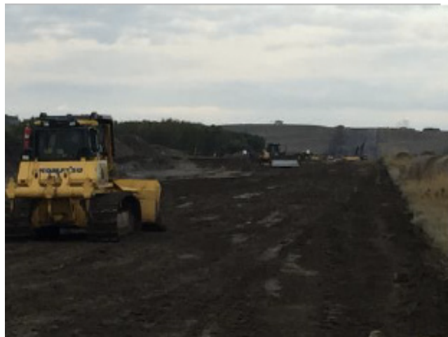
Dozer shaping subsoil – SF 37 – Sept 20, 2018
