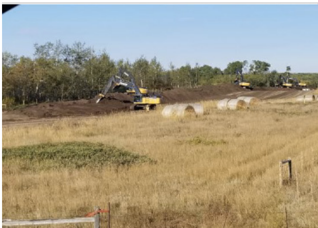
Excavators bailing topsoil – SF 32 – Sept 19, 2018
