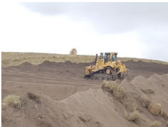
Dozer shaping and contouring – SF 32 – Sept 20, 2018
