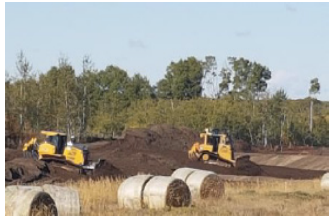
Dozer pushing topsoil on ROW – km 50+450 - Sept 19, 2018
