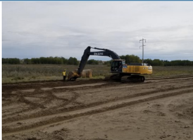
Excavator pulling roach - SF 28 - Sept 20, 2018
