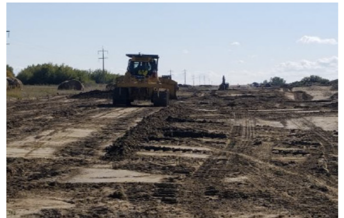
Dozer pushing topsoil on ROW – km 50+450 - Sept 19, 2018
