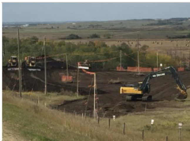
Dozer spreading topsoil and excavator working on roach – Sept 20, 2018
